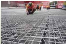
Glass Fibre Reinforced Polymer (GFRP)
