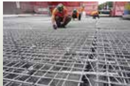
Glass Fibre Reinforced Polymer (GFRP)
